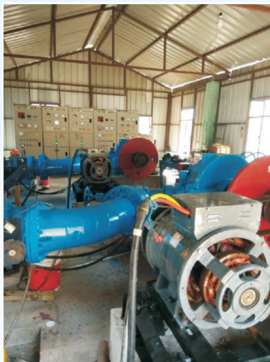
Plate 4: TG Set with control panels inside the Power House
