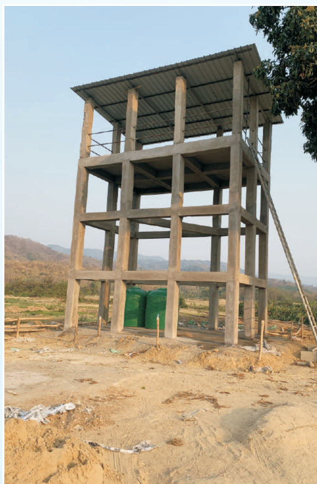
Plate 8: Overhead water tank for cleaning Solar panels
