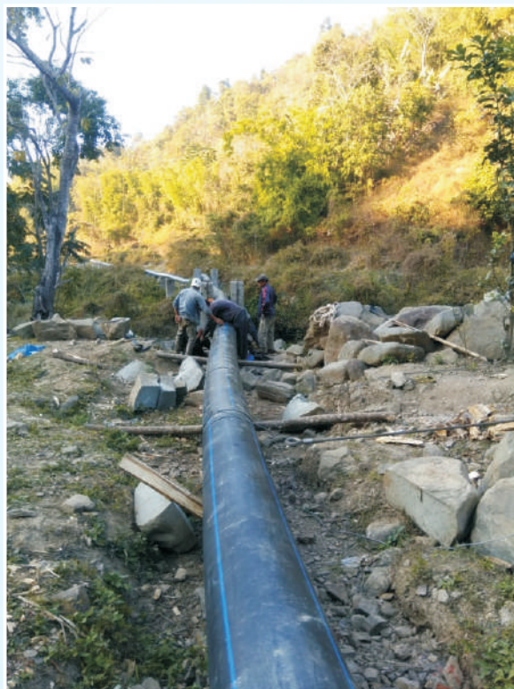
Plate 5: Laying of penstock pipe
