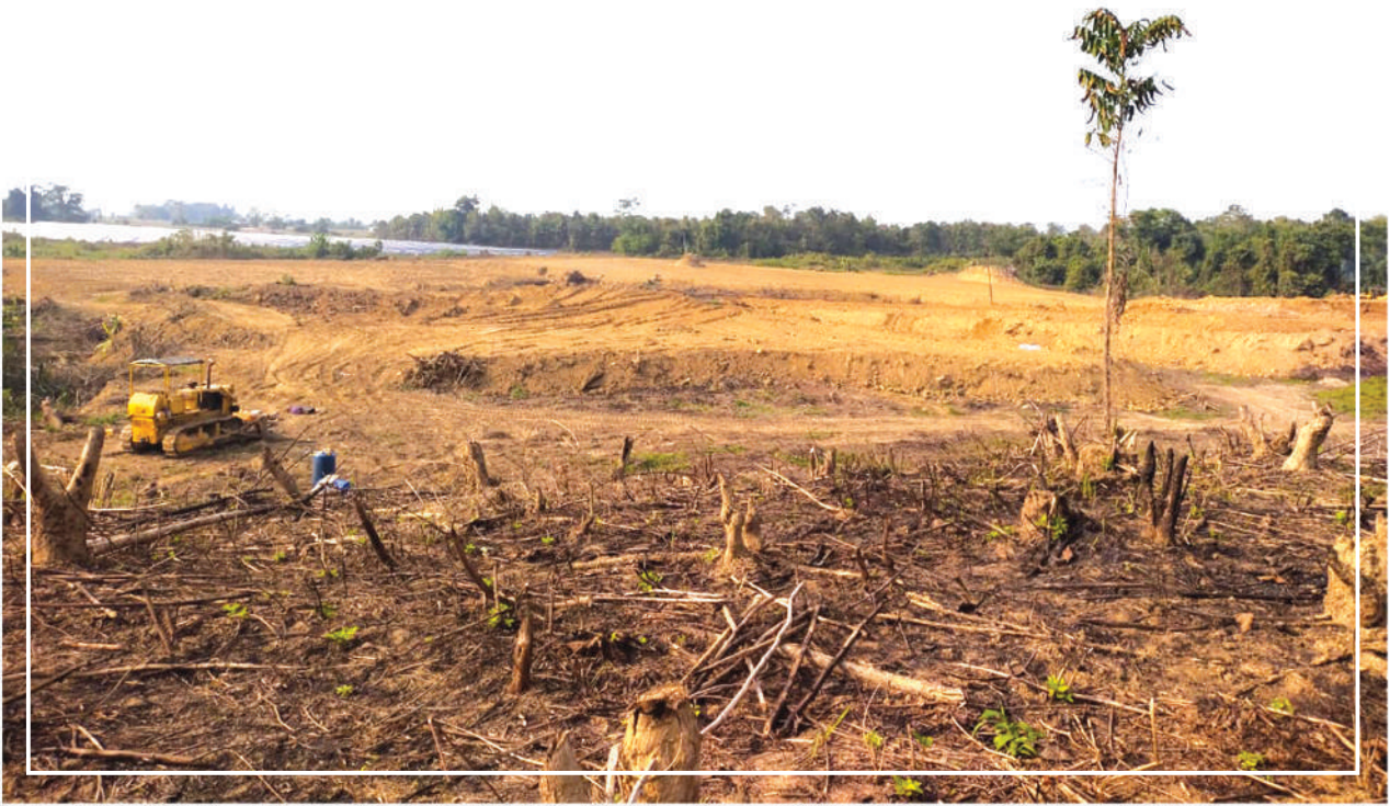
Plate 6: Site leveling under progress for phase –II 5MW Solar Power Plant at Hovukhu Village
