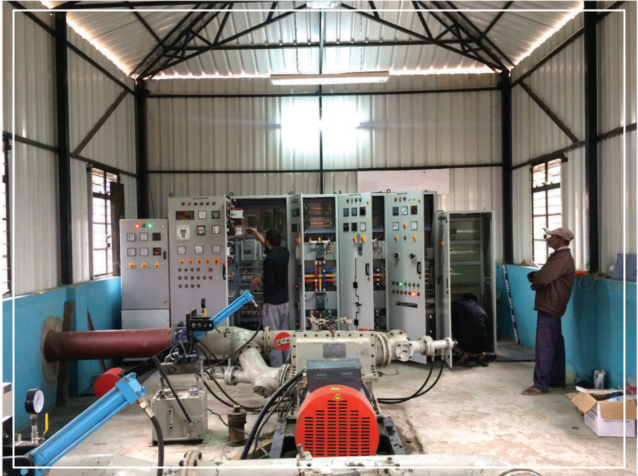
Plate 1: TG Set with control panels inside the Power House.
