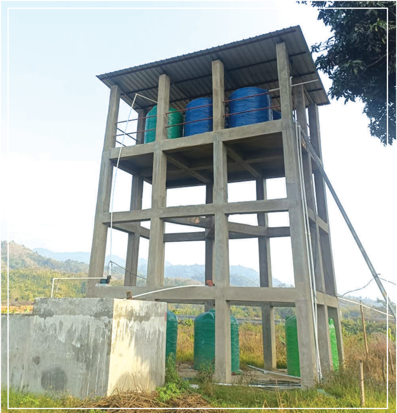
Playe 5: Over head water tank for cleaning solar panels of 5MW Solar Power Plant at Hovukhu Village
